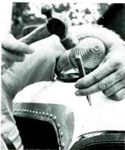
Fig. 4 Mark the spot for the hole (needed to bring the cable to the outside) by denting the roof with a centerpunch inserted in the access hole from the inside. Then, on the outside of the cab roof, centerpunch near the dent, and drill the 1/2-inch hole.
