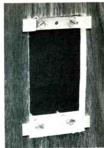
Fig. 4 Plaster straps are best for use on wallboard that's already there. Two strips at the top and two at the bottom clamp the wallboard between them when the screws are tightened. No stud is required.
